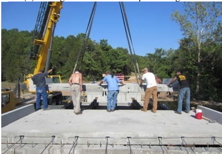
(c) Placing second concrete deck slab
