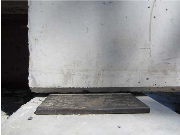
Figure 5.16: Bridge girders seated on a rubber pad
