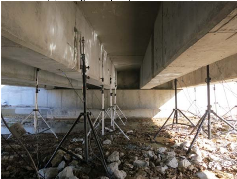
(c) Concrete-girder span (20 DC-LVDTs)
