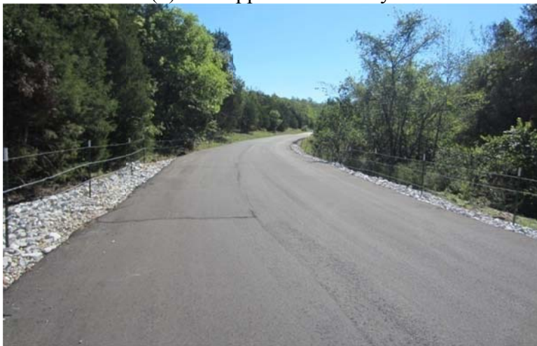
(c) West approach roadway
