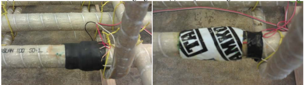
(g) Cover gauges and joints with additional rubber tape
