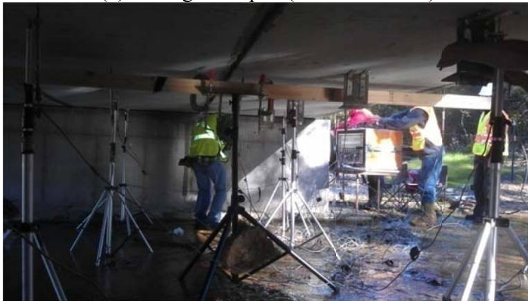
(b) Box-girder span (20 DC-LVDTs)
