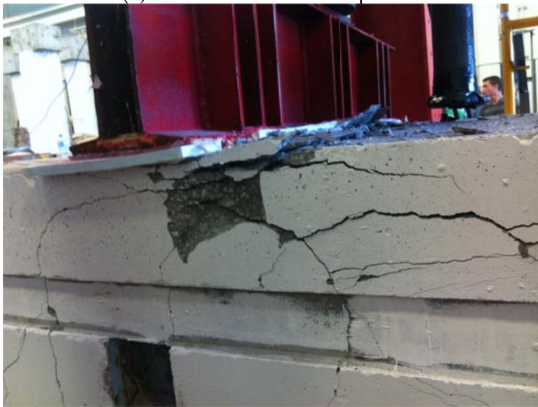
(b) Concrete crushing and horizontal splitting cracks
