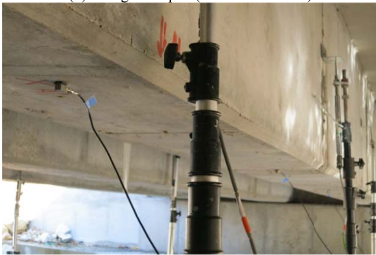
(c) Concrete-girder span (7 accelerometers)
