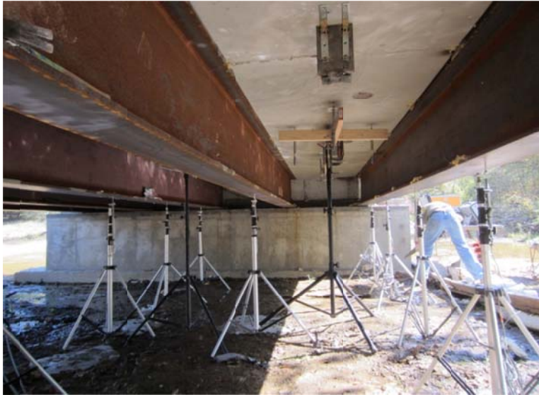
(a) Steel-girder span (20 DC-LVDTs)
